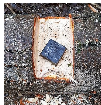
Figure 2: Rebar with a metal plate at one end, hammered through a log into the ground. A section has been removed from the log to ensure fixing is recessed (SFI).
